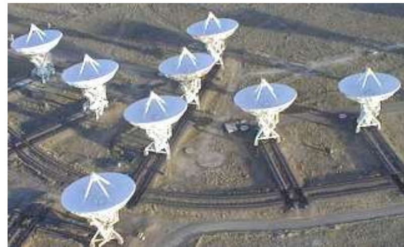
Parabolic surfaces: eliminate spherical aberration
